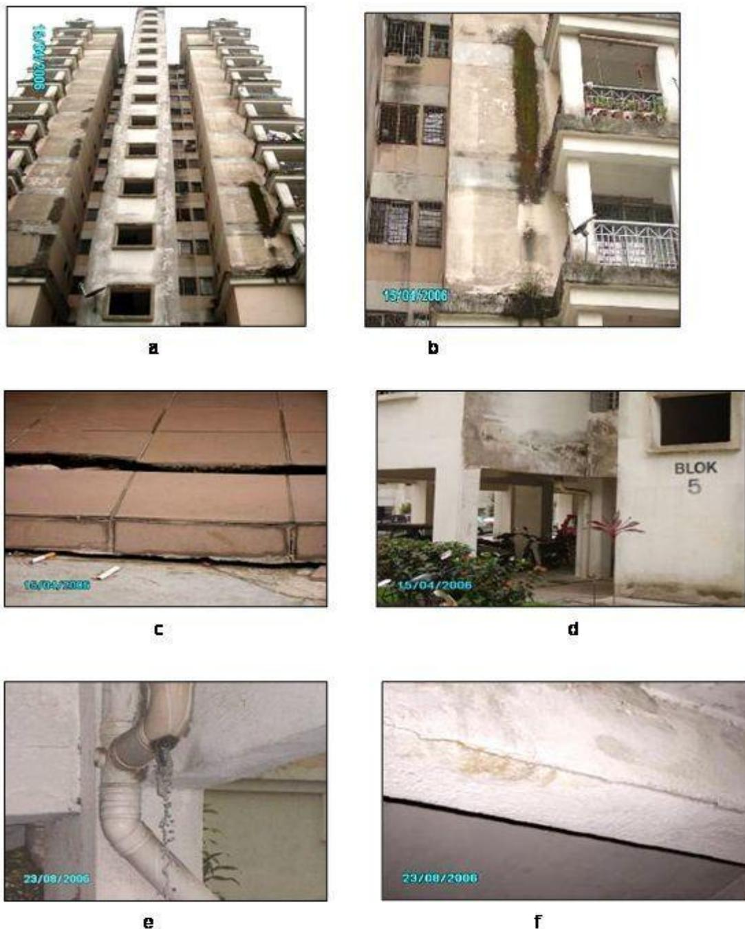
**Figure 3.** Façade and services defects at post occupational stage.
