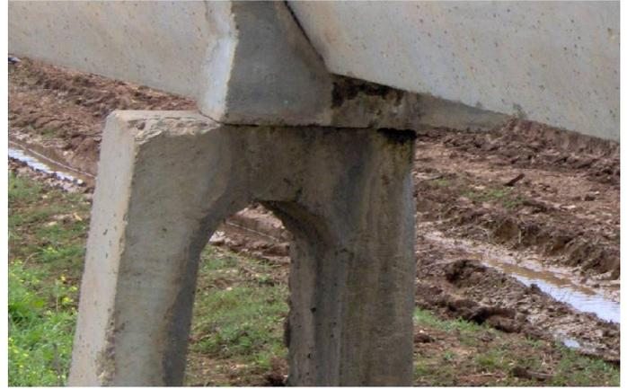
**Figure 4.** Sliding of supports at canalette.
