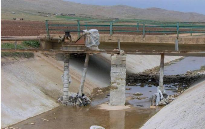
**Figure 5.** Unauthorized water outlet at Urfa main canal.
