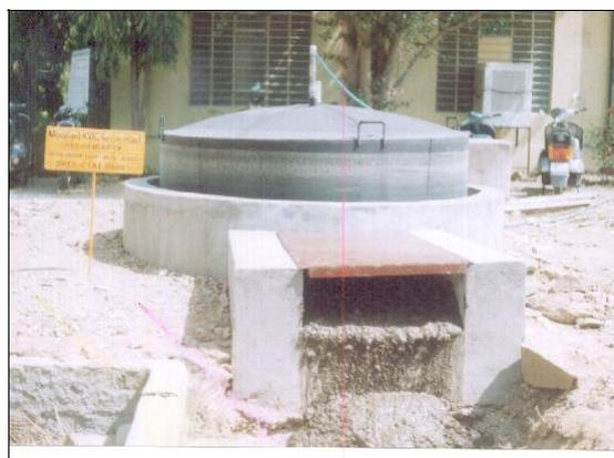
**Figure 4.** *Jatropha* based biogas plant (floating drum type).
